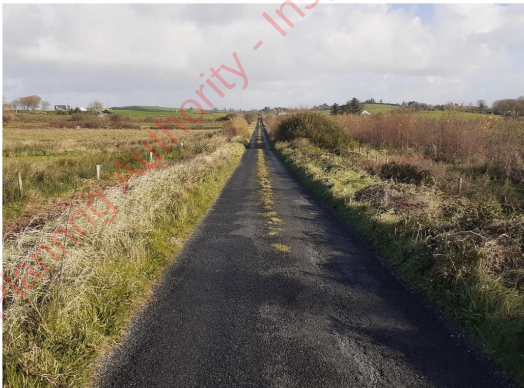
Plate 6.26. View of section of L6132 local road where hedging is largely absent - looking eastwards (November 2023).
