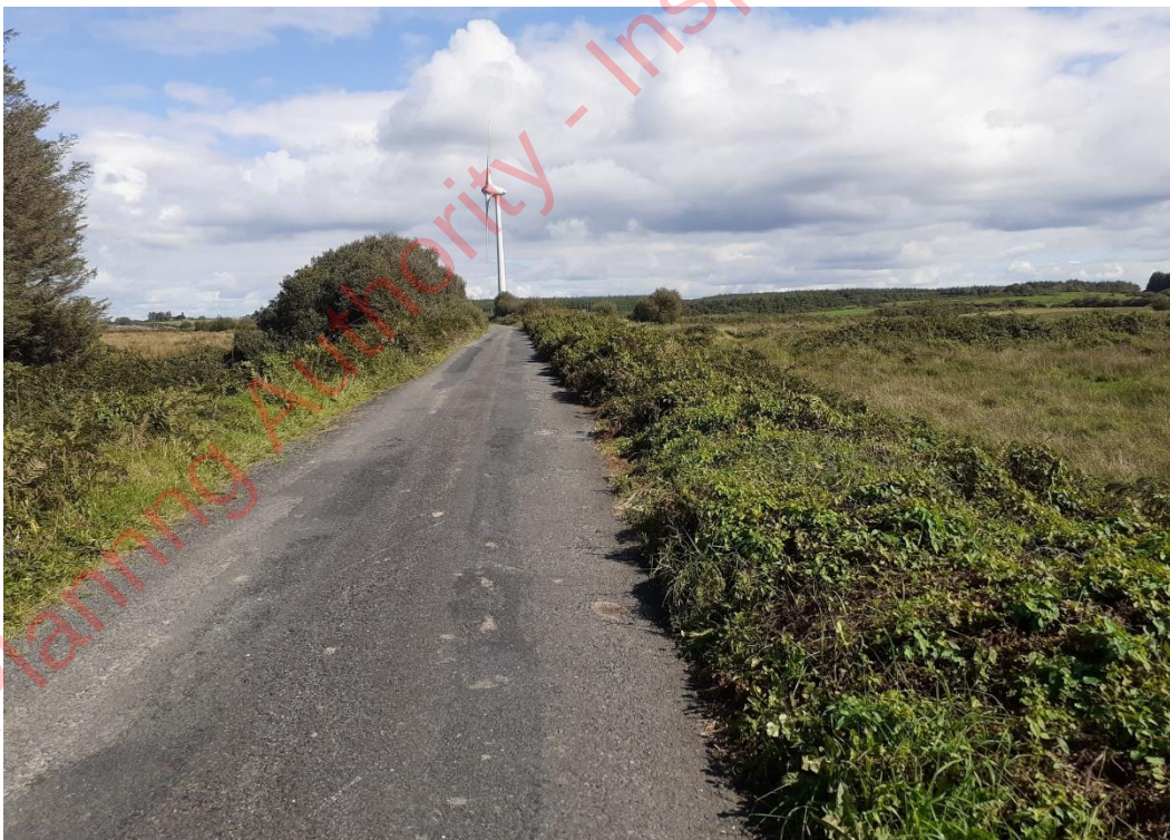
Plate 6.24. View of local road running eastwards towards Tullabrack 110kV Substation. This section is lined by scattered hedging and low banks often dominated by bracken and brambles – looking eastwards towards Moanmore Wind Farm (September 2023).
